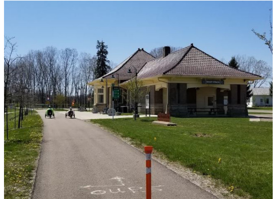
Example of CA&O Depot repurposed into trailhead and visitor center, Kokosing Trail, Mt. Vernon, Ohio.
