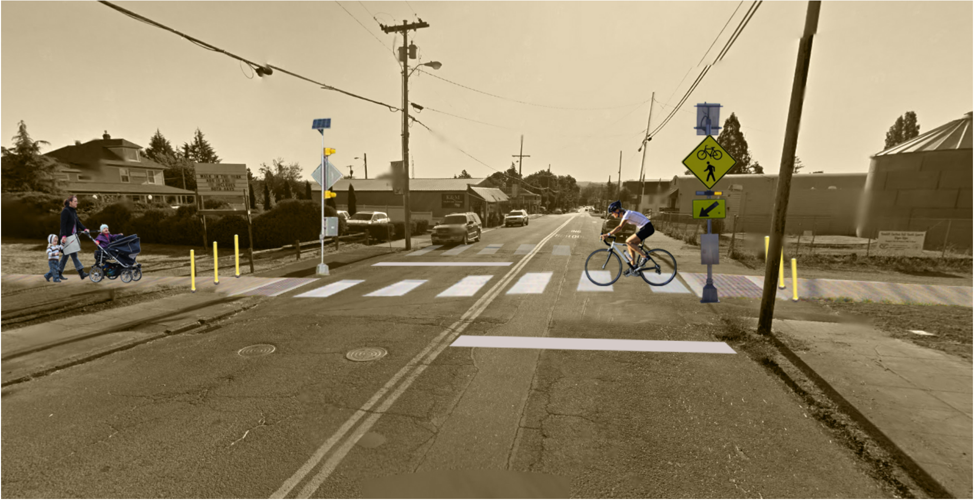
An artist rendering of a typical safe road crossing that includes a dedicated crosswalk, pedestrian activated flashers, signage, bollards, a change of material where the trail meets the road, and set-back vehicle stop lines.
