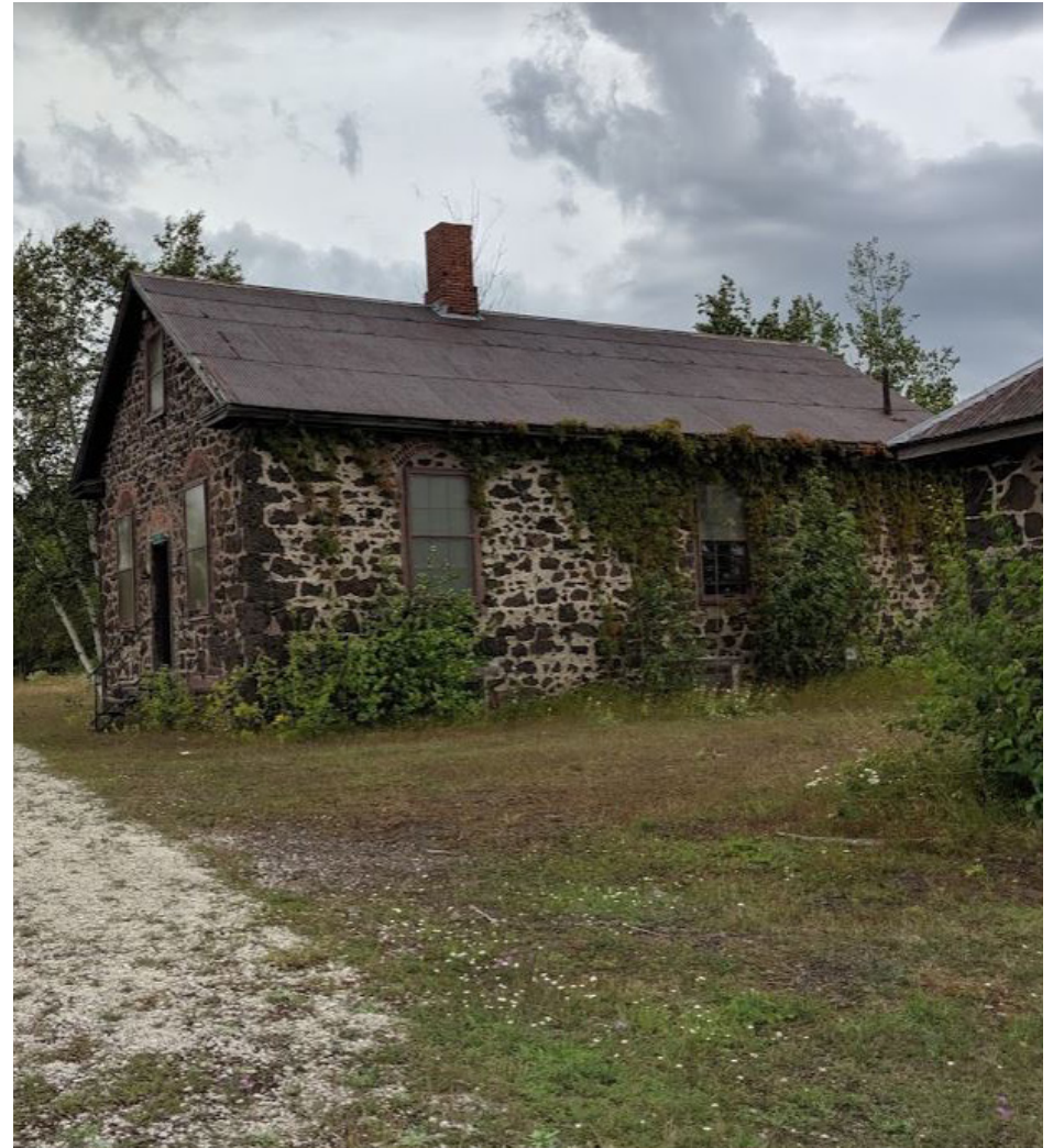
The Calumet and Hecla Mine Captain's Office. Calumet, Michigan.
