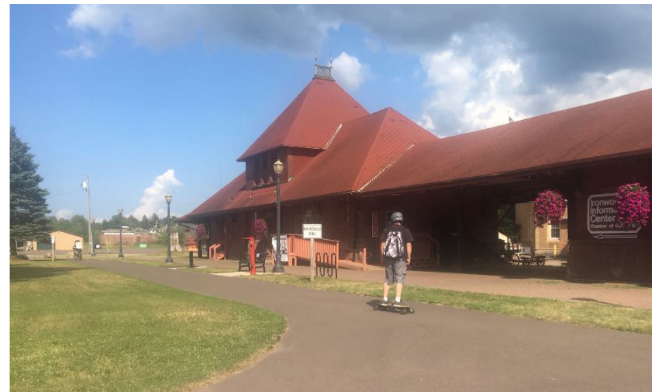
Top Photo: The historic Calumet Railroad Depot is shown above.
