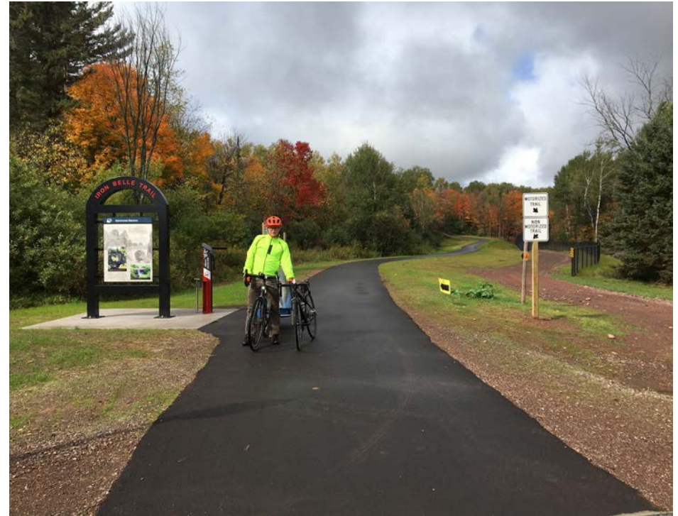
Separated and parallel trails on 3-mile Bessemer to Ramsey Section of the Iron Belle Trail.
